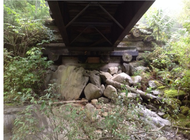
Right Bank Abutment when facing downstream
