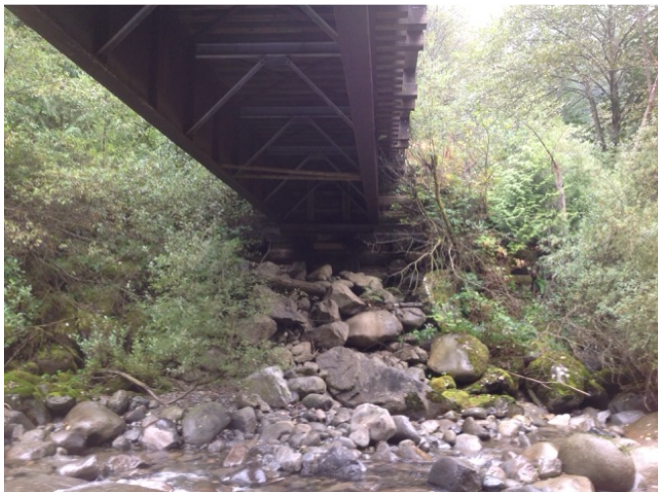
Left Bank Abutment when facing downstream
