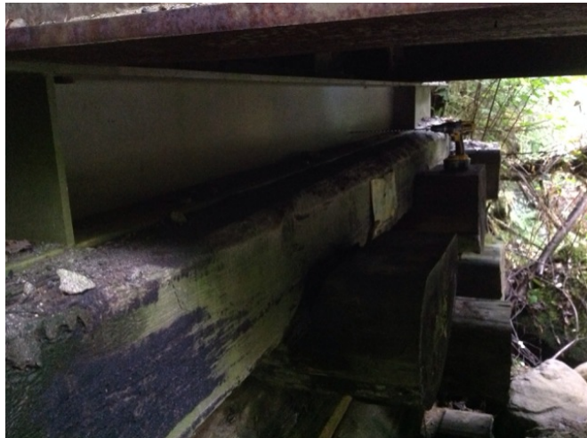
left bank bearing
